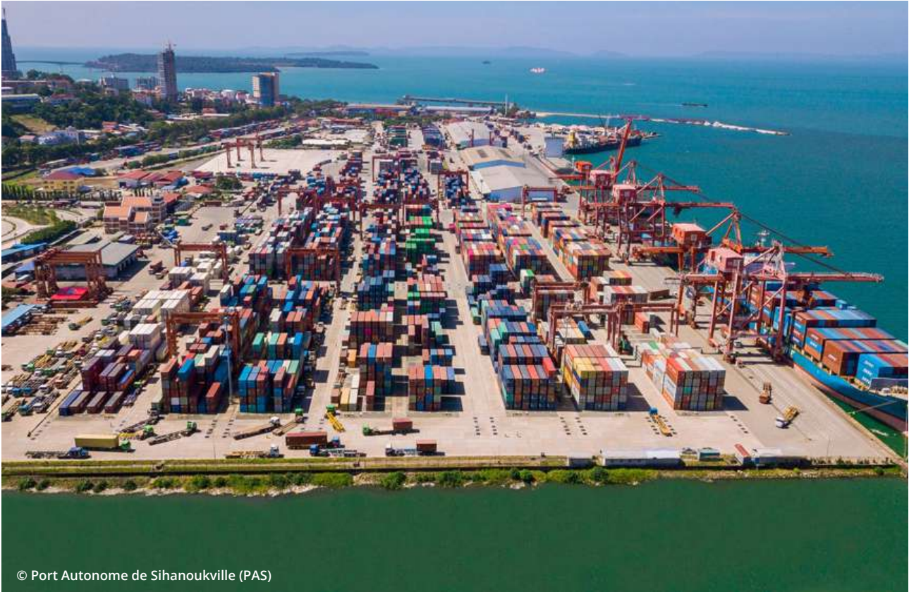
Aerial Photograph of Sihanoukville Autonomous Port
